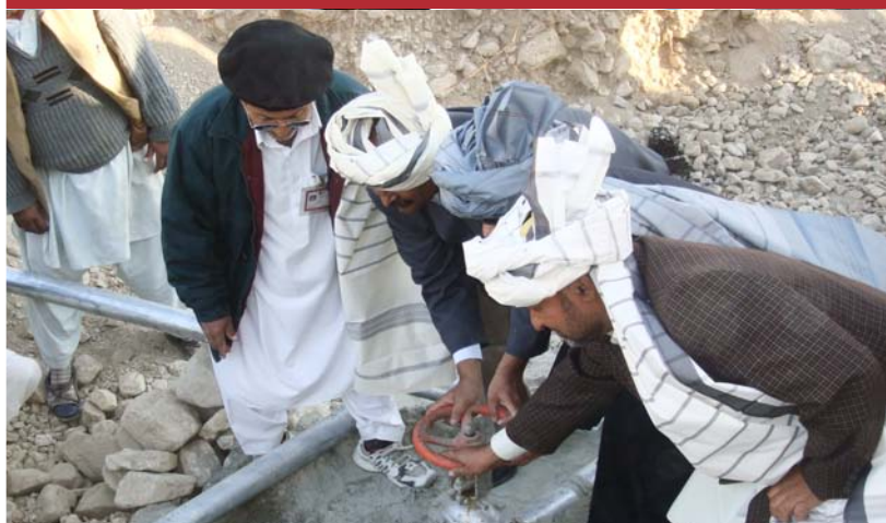
Water Supply Scheme at Pezu
